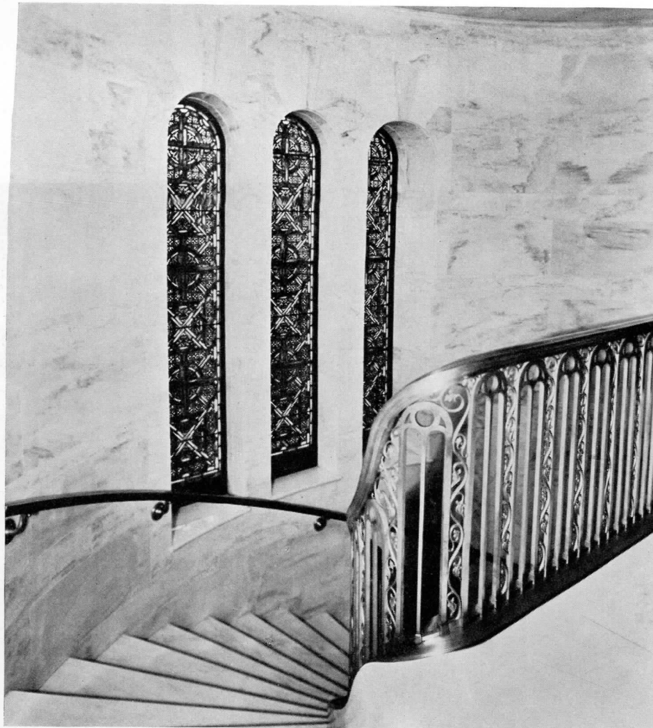
Looking down from the head of the stairs, Mayfield Mausoleum. Note the beauty of the curved pieces of wall and window soffits, which fit perfectly.
