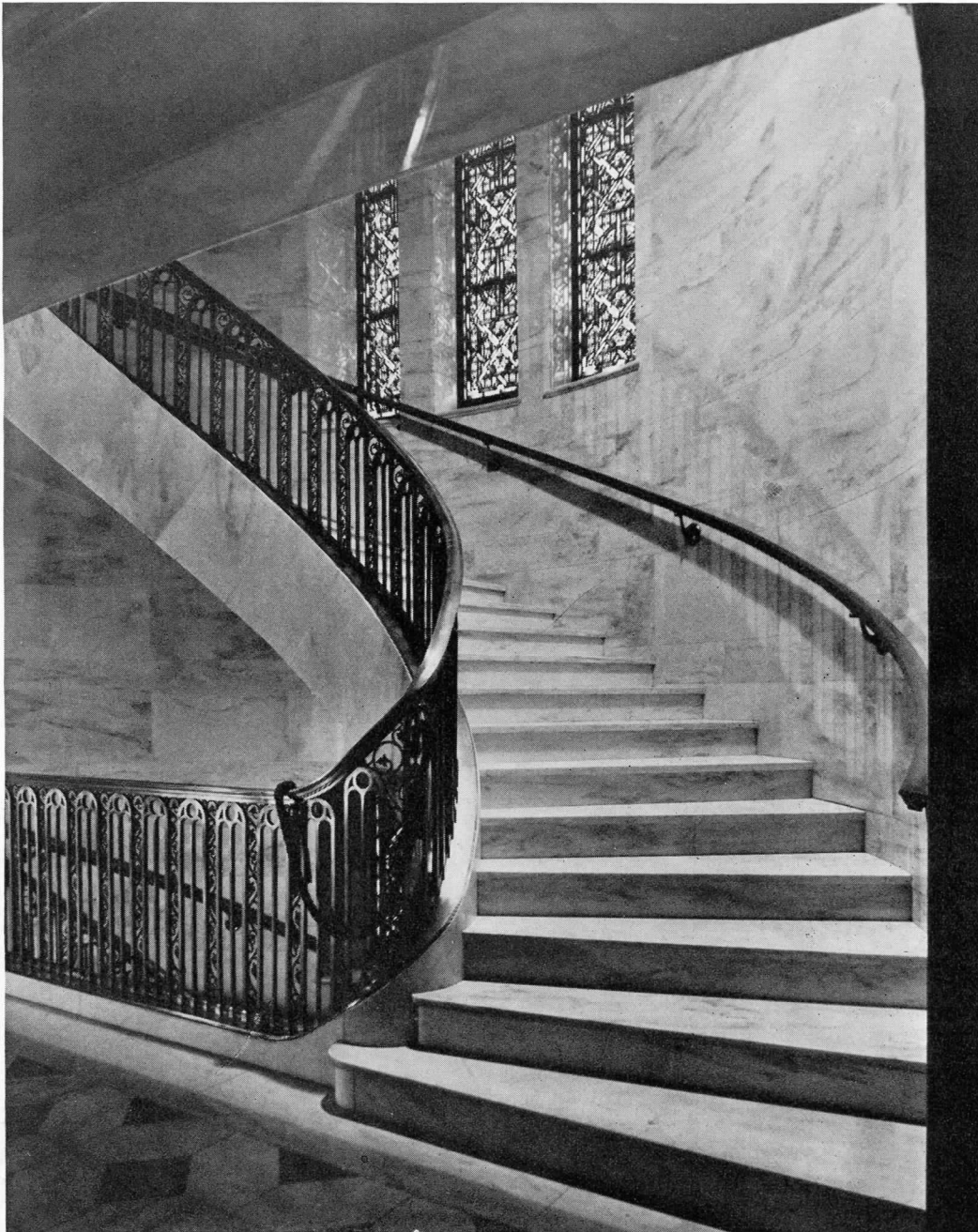
Stairway of Alabama marble, from chapel floor to second floor, in the Mayfield Mausoleum, Cleveland.
